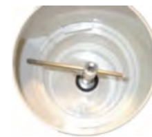
Hold plugs in place for vacuuming
