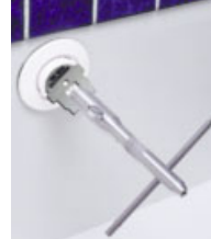
3. Install/remove directional wall fit- tings
